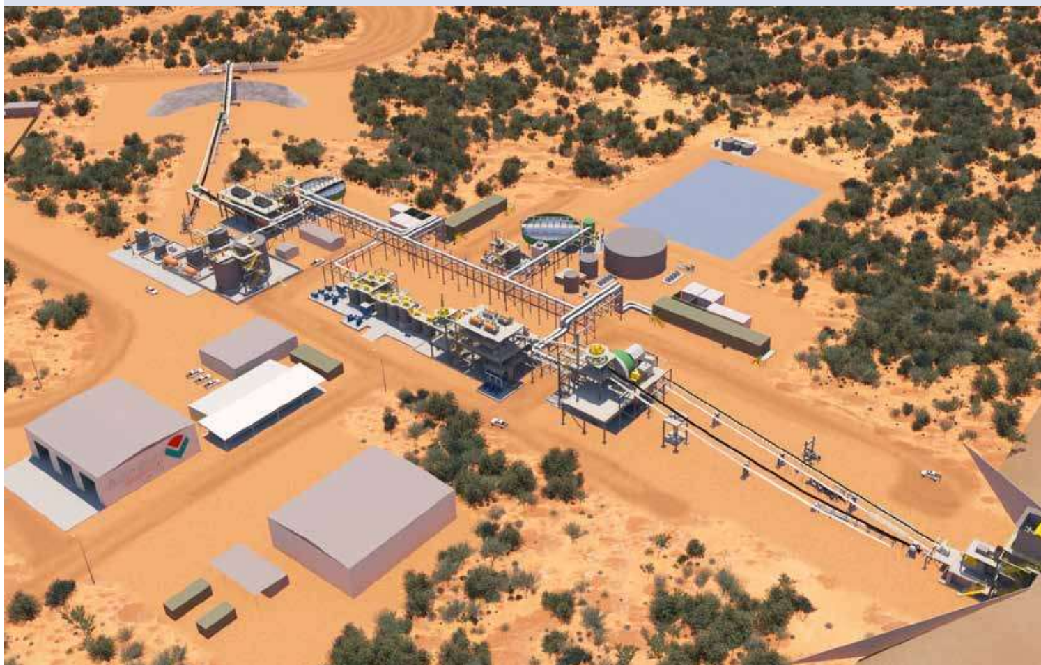
Australian Vanadium has engaged Primero as a contractor for early works on the planned processing plant at its namesake project in WA
